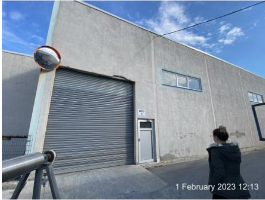
Outside view of B5 Dyeing.JPG
