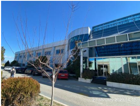
Building 1 main management and sewing.JPG
